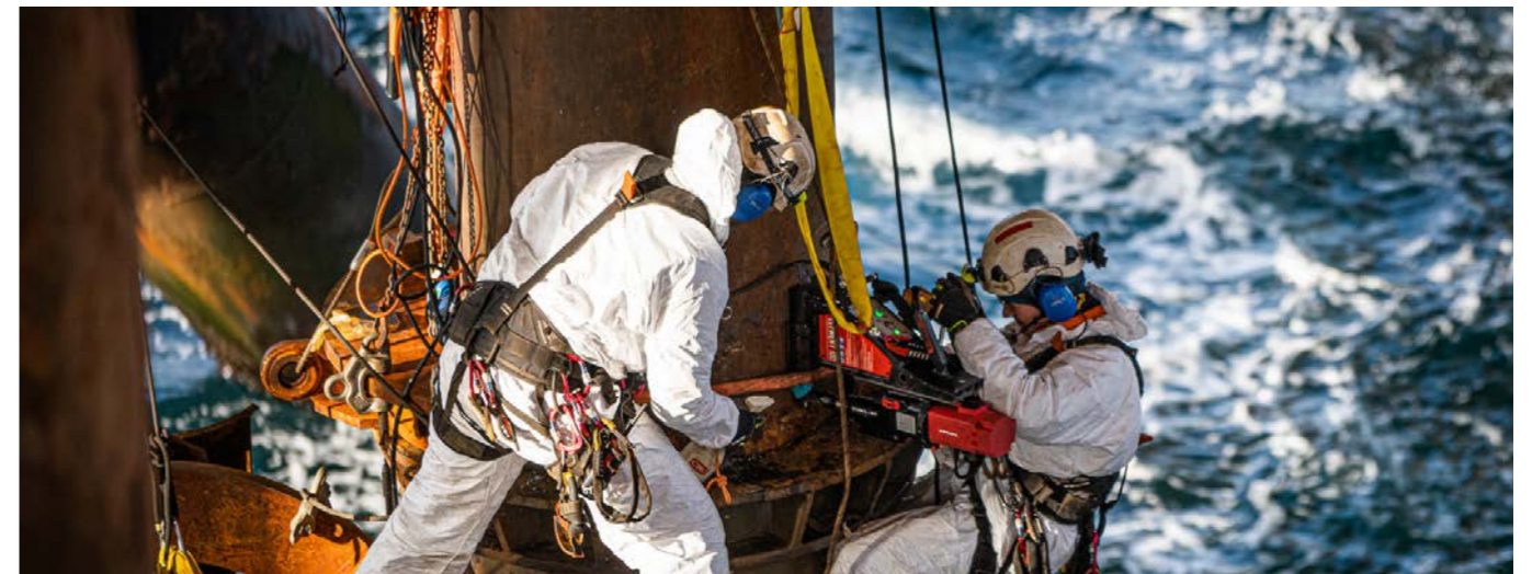
Gyda decommissioning and completion of preparation phase.
